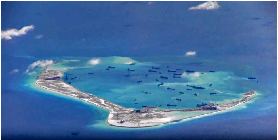
Example of the construction of a Chinese military fortification on an artificial sand island in the South China Sea. (Source: U.S. Navy.)
