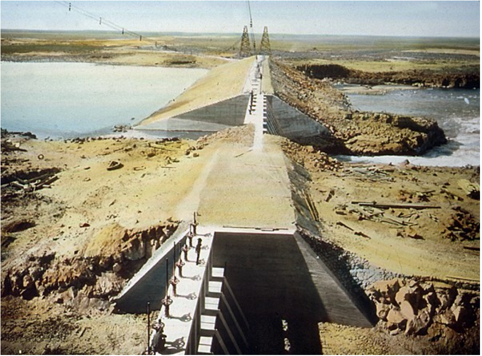
Figure 7: Minidoka dam being built.
