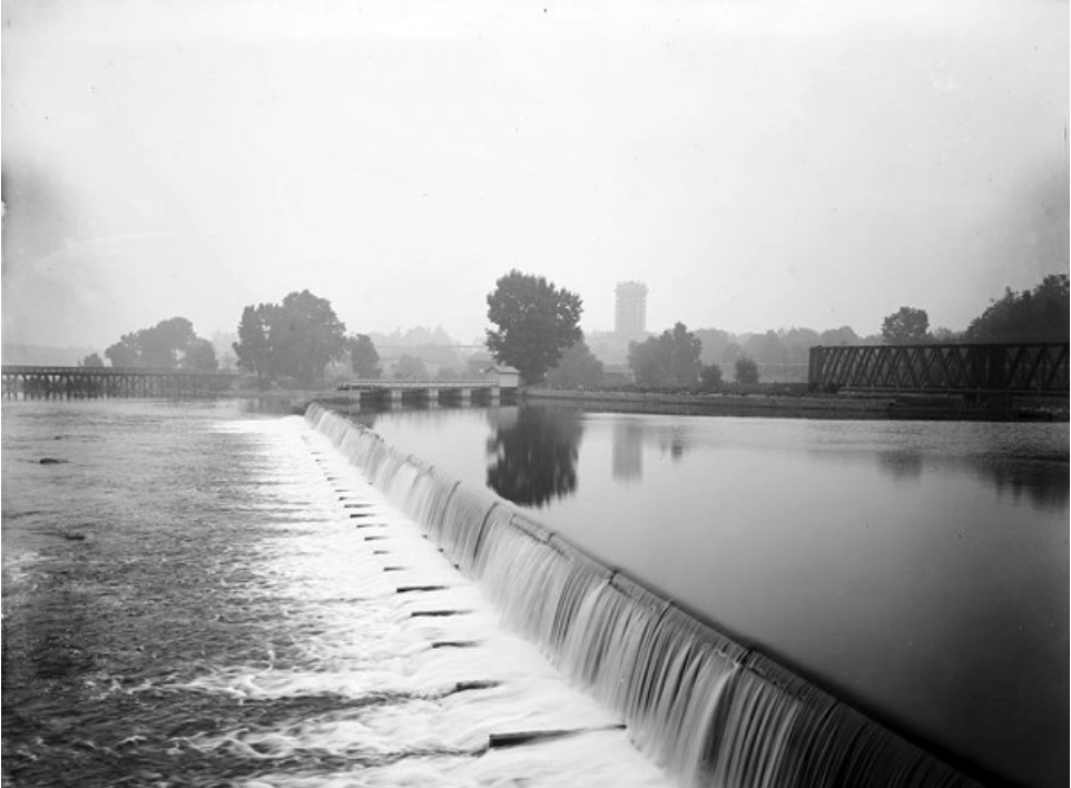
Figure 5: The site of the first American hydroelectric dam built on the Fox River at Appleton, Wisconsin in 1882.
