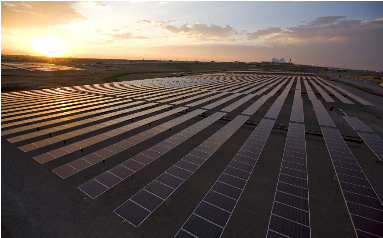
Figure 15: Solar farm using 1-axis tilting photovoltaic panels. This farm is located at the Denver International Airport. Note that the ground is cleared and leveled. (Credit: National Renewable Energy Laboratory for the U.S. Department of Energy, used as permitted.)
