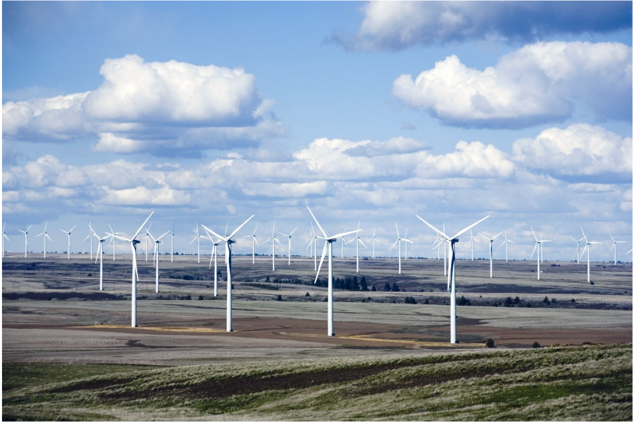
Figure 17: Wind farm in Washington. These wind turbines are closely spaced in rows to handle prevailing winds primarily from one direction. These turbines have a hub height of only about 60 m compared to turbines with hub heights up to 140 m used in this analysis. (Credit: Mike McPheeters, National Renewable Energy Laboratory for the U.S. Department of Energy, used as permitted.)
