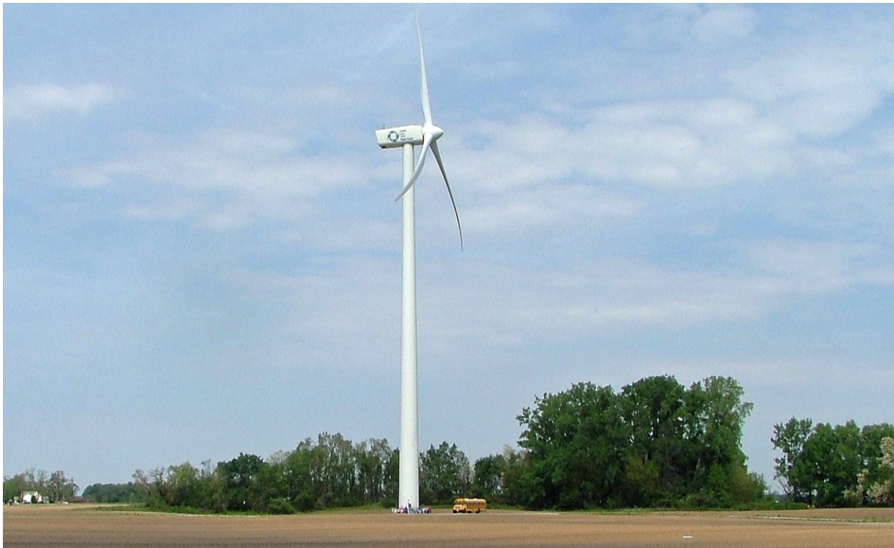
Figure 11: School bus next to a wind turbine with a 79-m hub height. Most wind turbines would have hub heights of 110-140 m with 100+ m diameter rotors. (Credit: J.M. Snead.)
